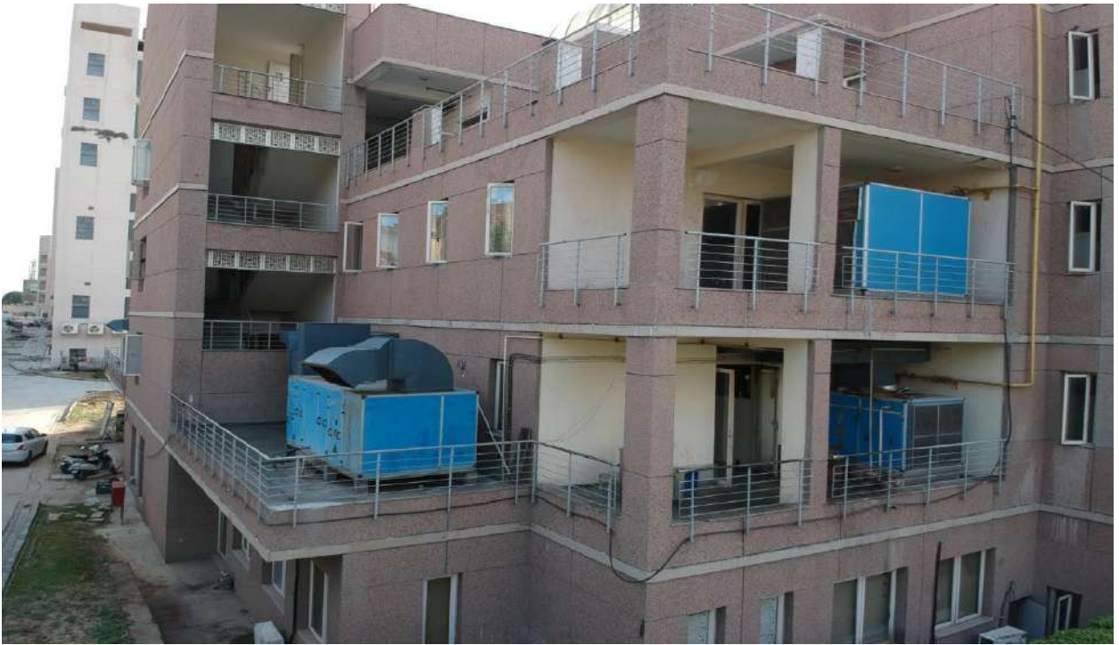
Air Filtration Unit
