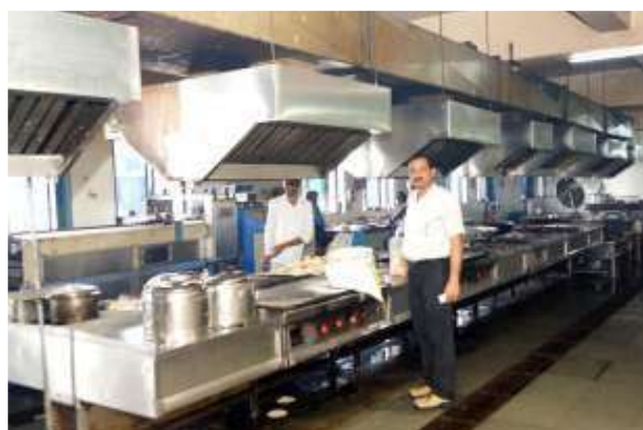
Cooking Area and Chimney
