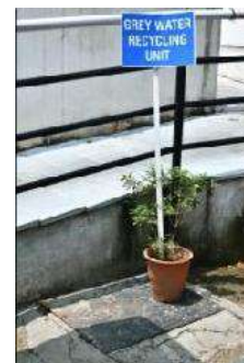
Grey water recycling unit
