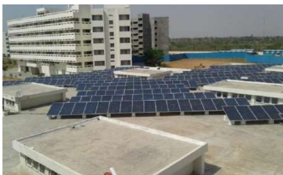
Solar panels of 1.8 MW capacity installed at SIUs' Lavale campus as renewable energy source.
