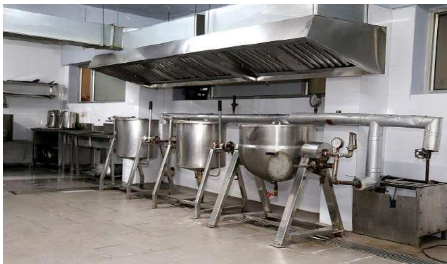
Kitchen Area with Chimney
