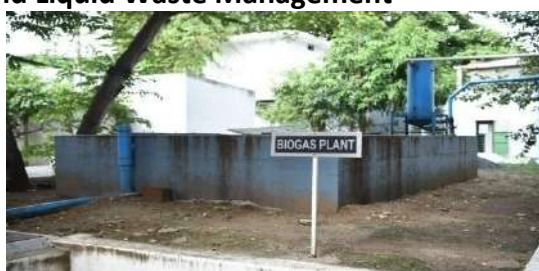
Bio Gas Plant
