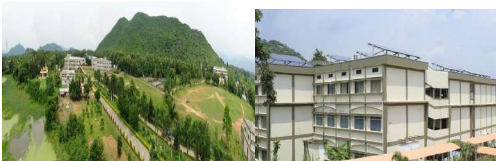
Solar Power Panels
