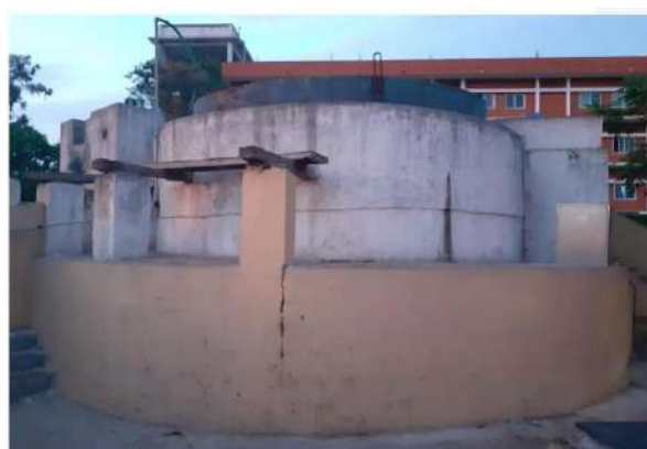
Solid Waste Management –Bio Gas Plant
