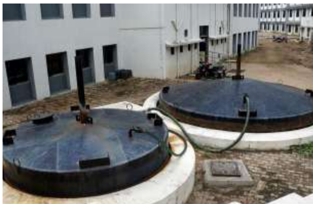
Functional Biogas Unit
