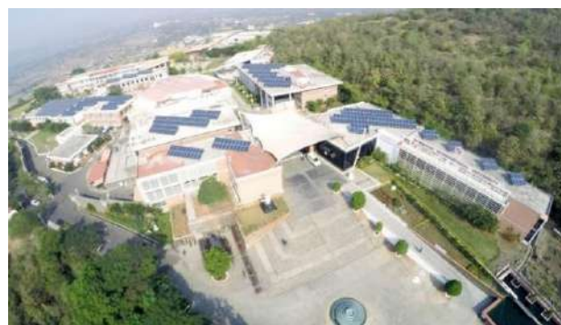
Solar panels of 1.8 MW capacity installed at SIUs' Lavale campus as renewable energy source.
