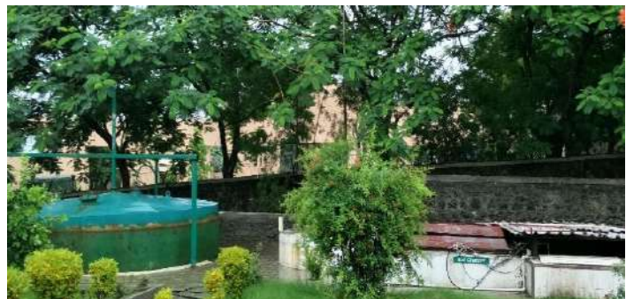
'Nisargruna' Biogas plant of 1 TPD capacity
