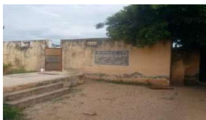
Before Intervention – Damaged School Toilet Complex
