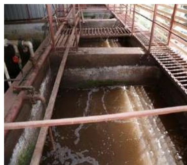
Liquid waste treatment
