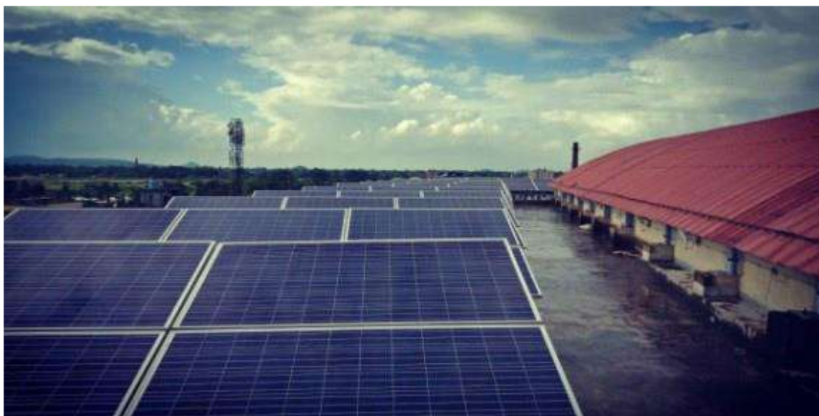
Roof-Top Solar Photo Volatic system
