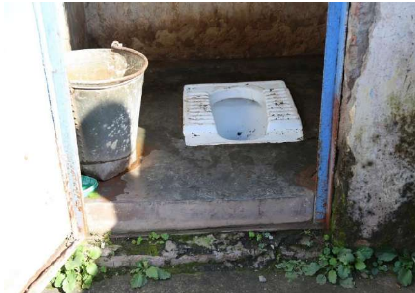
Toilet in Village Barog Pre-Cleaning
