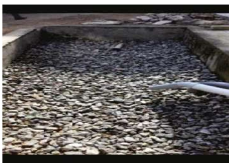
Water is stored by the rain water harvesting method
