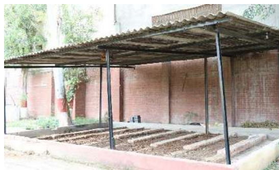
Vermi Compost Pit
