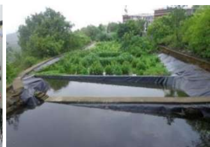
Reed bed for wastewater treatment
